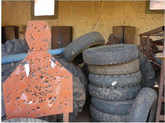
Images of the lodge destroyed by the LRA in the January 2, 2009 attack on Garamba National Park headquarters
